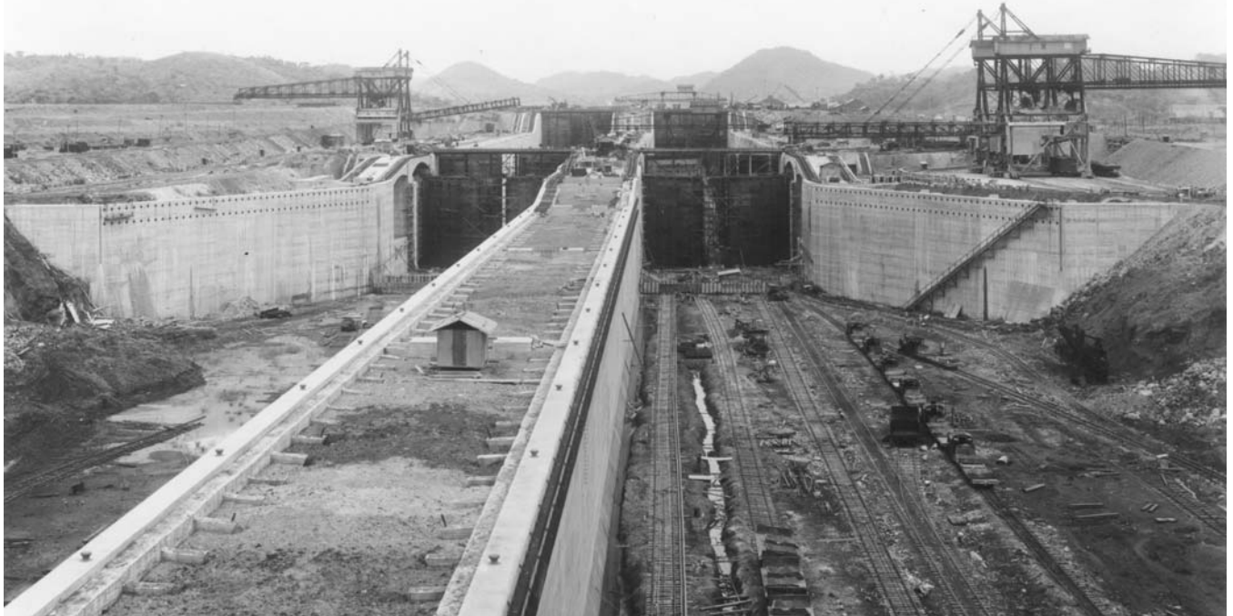
Miraflores Lower Locks During Construction, June 1913
